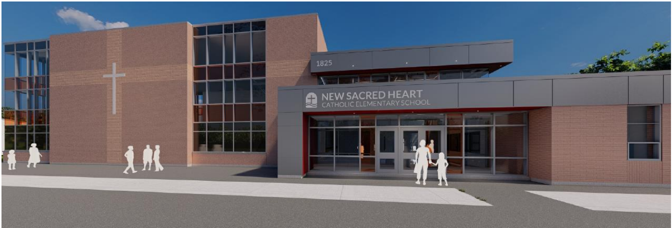
Exterior of renovated main entrance design
